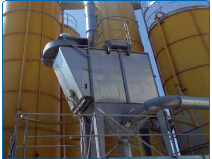
WEIGH HOPPER INSTALLATION
